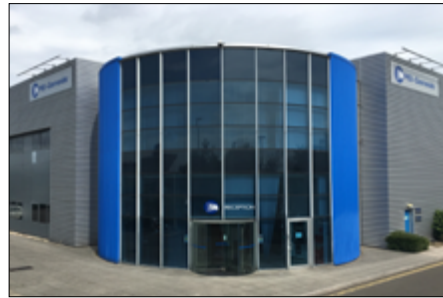
European Headquarters & Production Facility, Southampton, UK
